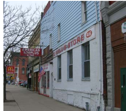
Poorly maintained facade
