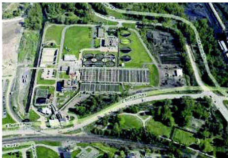
Erie Wastewater Treatment Facility
