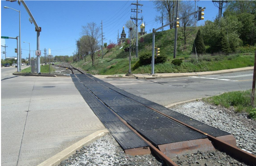
Photo 21: Looking east at CSX Railroad tracks.
