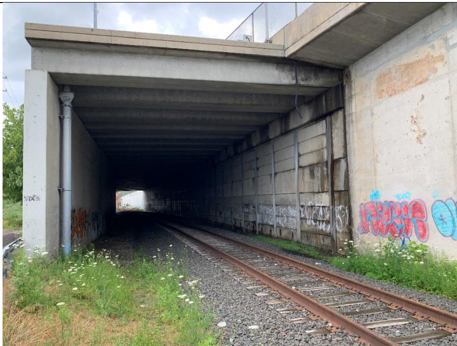
Photo 10: Looking east on Front Street towards abandoned CSX railroad.
