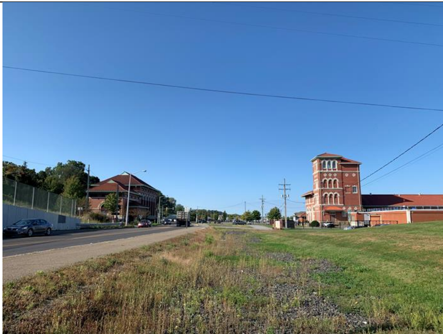
Photo 4: of Bayfront Parkway looking west, towards Chestnut Filtration Plant.
