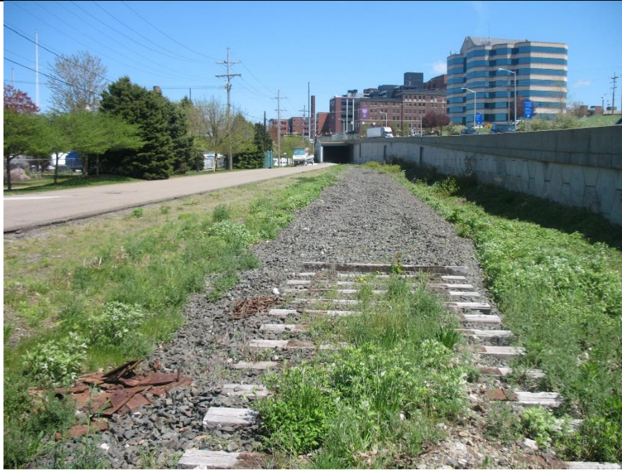
Photo 7: Looking east on Front Street towards abandoned CSX railroad.
