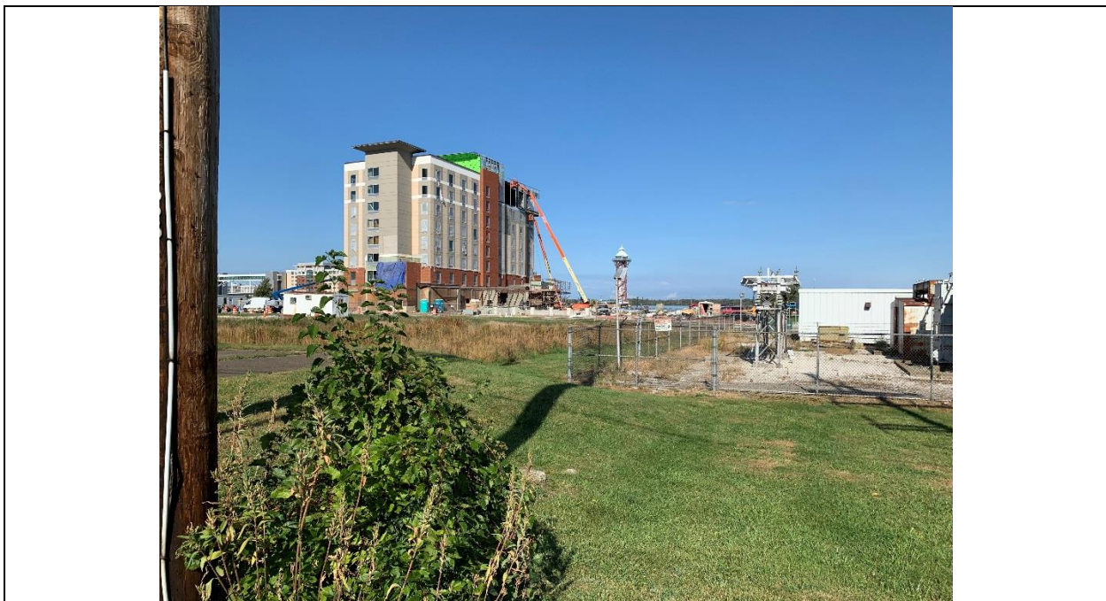
Photo 12: Looking at former GPU Front Street Station, now Hampton inn and Penelec substation.
