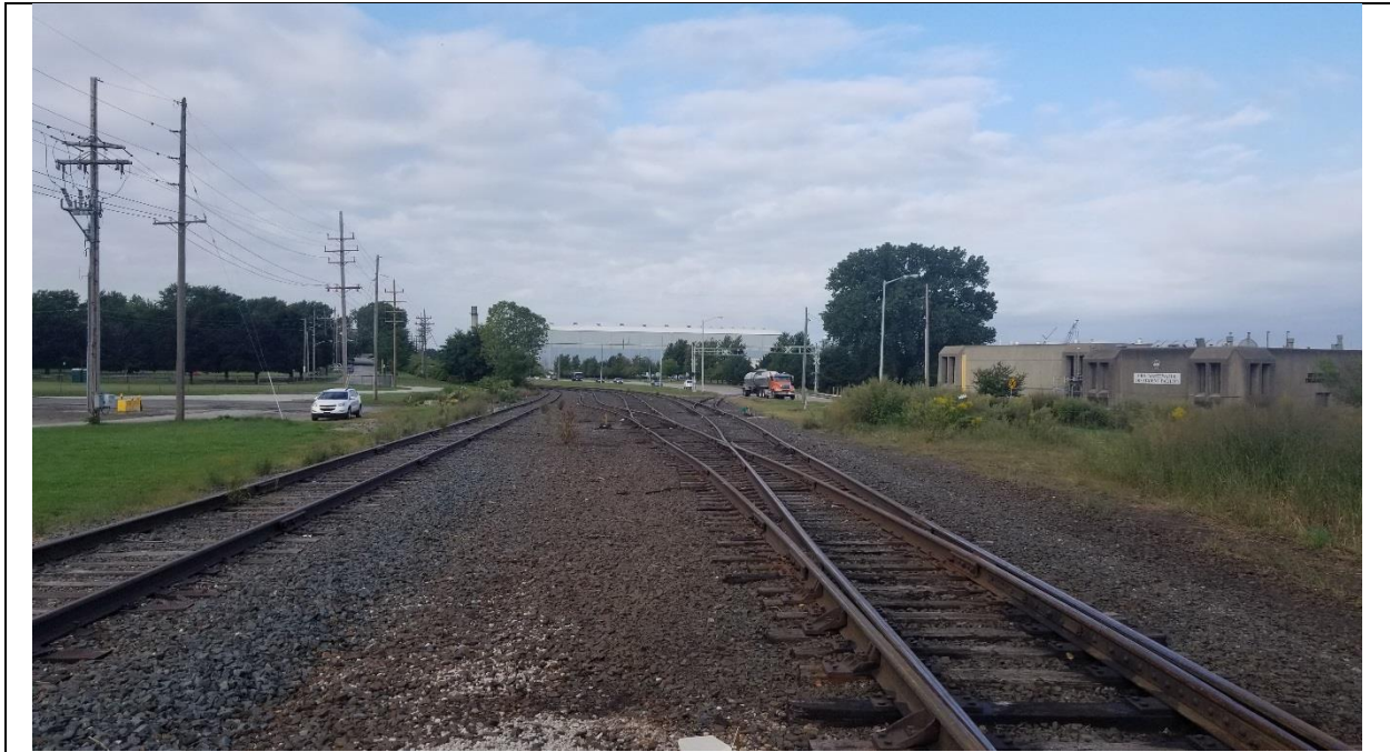
Photo 25: Looking north west at CSX Railroad tracks.
