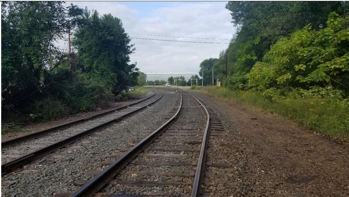
Photo 24: Looking north west at CSX Railroad tracks.
