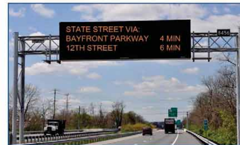
The 12th Street Signals Project also includes ITS signs on I-79 and the East Bayfront Parkway to provide real-time traffic information and weather conditions to motorists entering the City.
